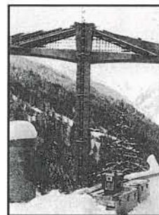
Vibration measurements of bridge supports
