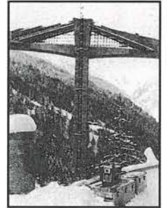
Vibration measurements of bridge supports
